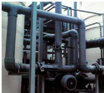
C-PVC pipes and moldings in the chemical industry
