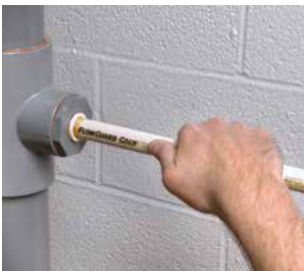
Installation of C-PVC pipes
